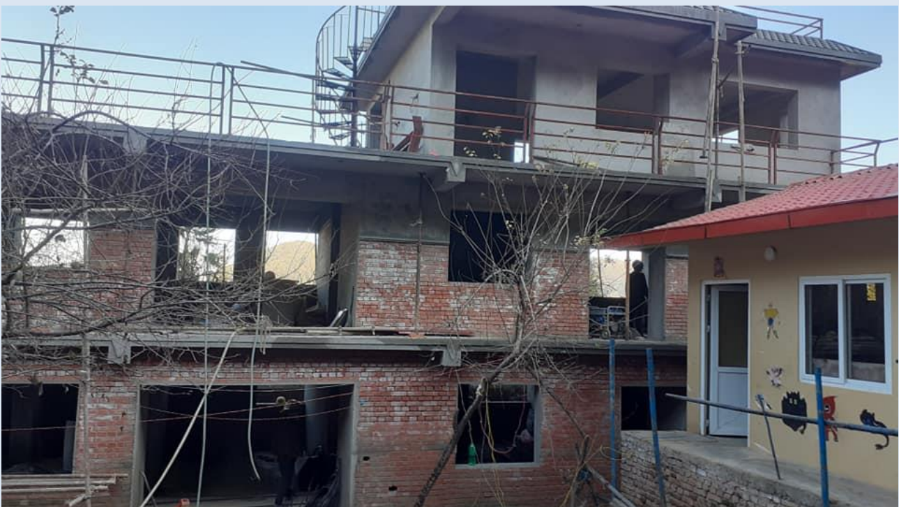
The new building in Godawari still under construction
